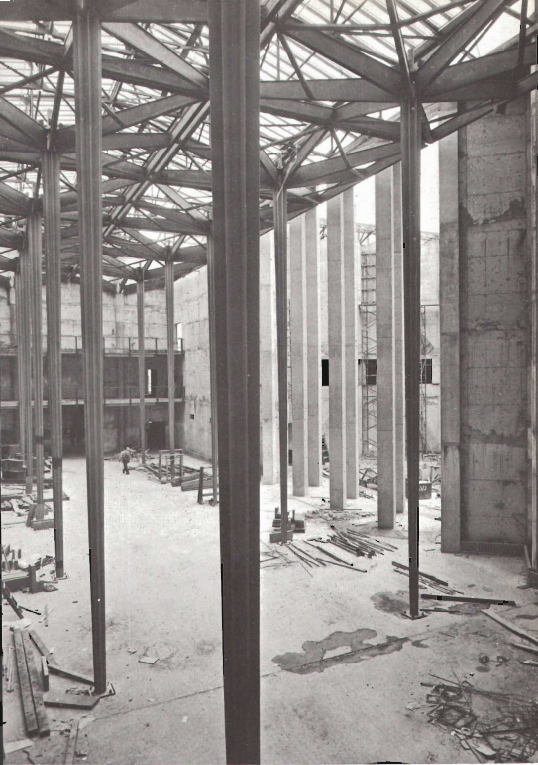
[National Gallery of Victoria Reception Hall under construction showing the framework for the stained glass ceiling designed by Leonard French.
