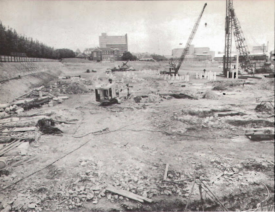
Clearing of the site for the foundation work.
